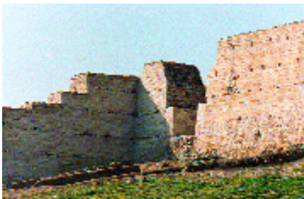
Muralla medieval de Alarcos restaurada
