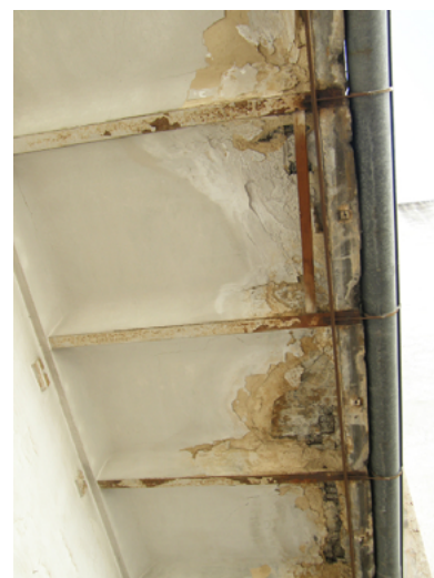
Image 8 | Structural view of a cantilever with narrow flange metal beams and wire-reinforced cement. Back façade of Gran Vía No. 27. Photo: Roser Martínez Ramos
